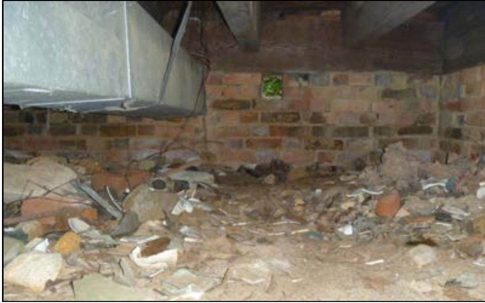
Artifacts in South Wing Crawlspace, facing East
