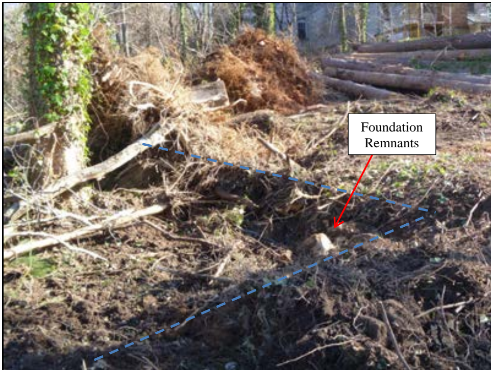
Approximate Location of Structure D, facing Northeast (after tree clearing).
