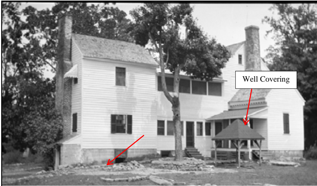
South Elevation, Crabtree Jones House [date unknown] Note Well House
