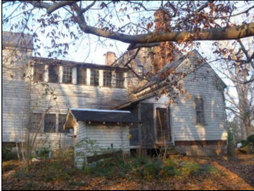
Well House (Structure E), facing North.
