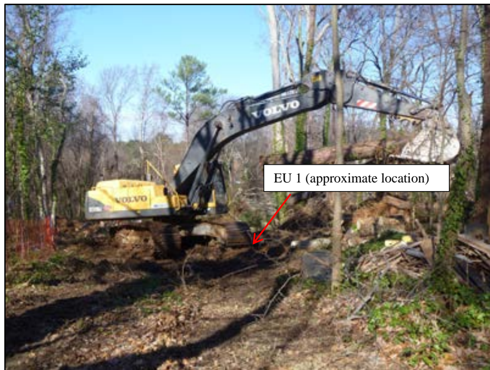
EU 1 (after Bulldozing).
