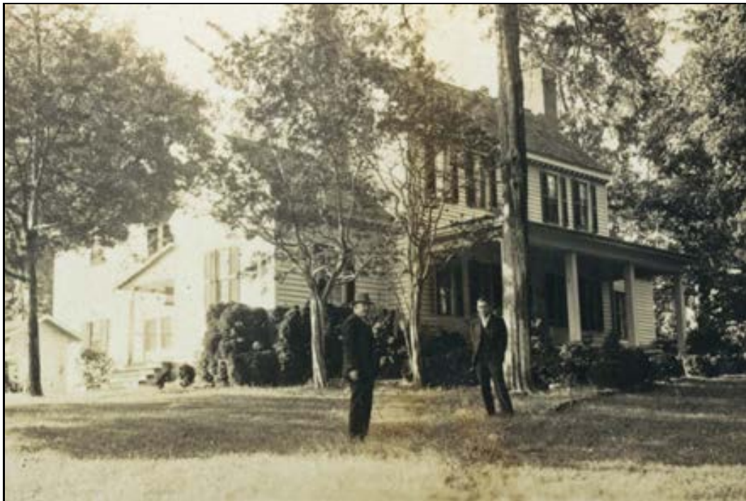
East and South Elevation, Crabtree Jones House [c. 1934] (Photograph by Frank Parker, Courtesy of Jones-Belvin Heirs)
