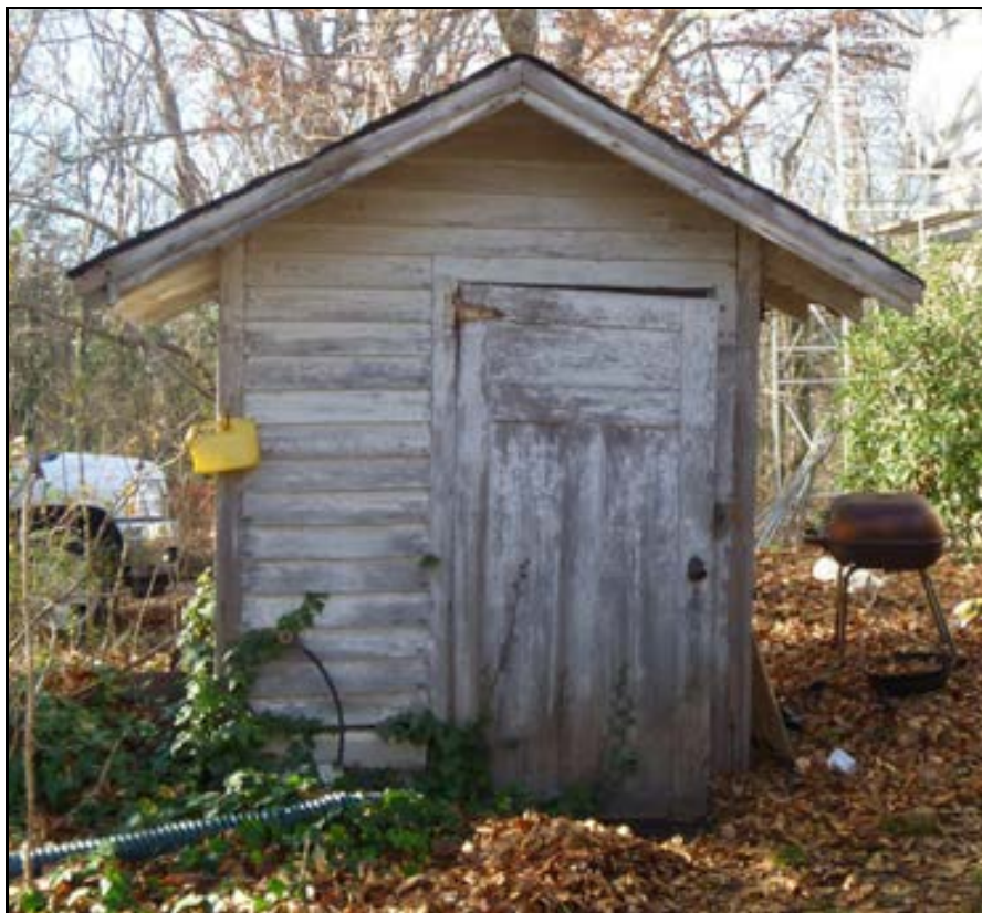
Well House (Structure E), facing West.
