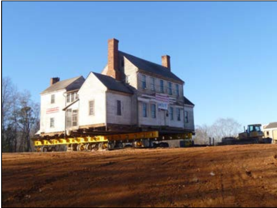
Crabtree Jones House, facing Northwest (January 2014)
